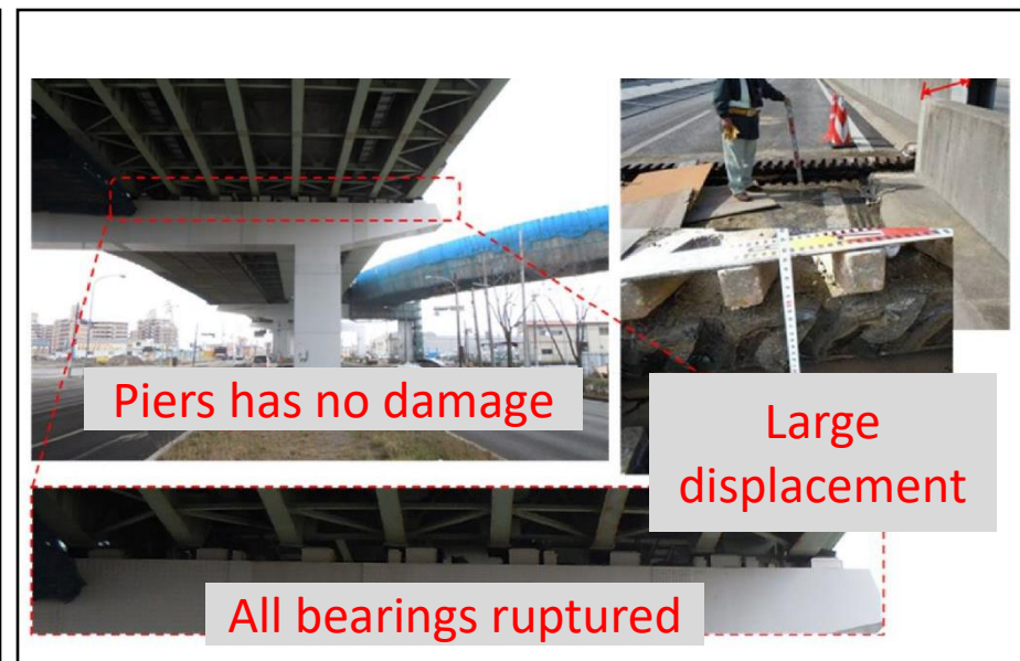
(JSCE, Steel Structure Committee)
